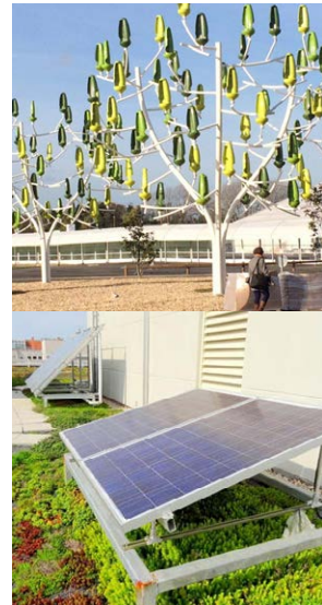
Photovoltaics installed on rooftops are a favorable solution to on-site energy generation (bottom). Micro wind production is less efficient but may serve educational purposes (top).
